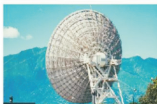
Communication base station
